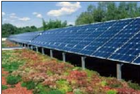
Figure 5.1: A Rooftop that is Both Green and Solar Powered
