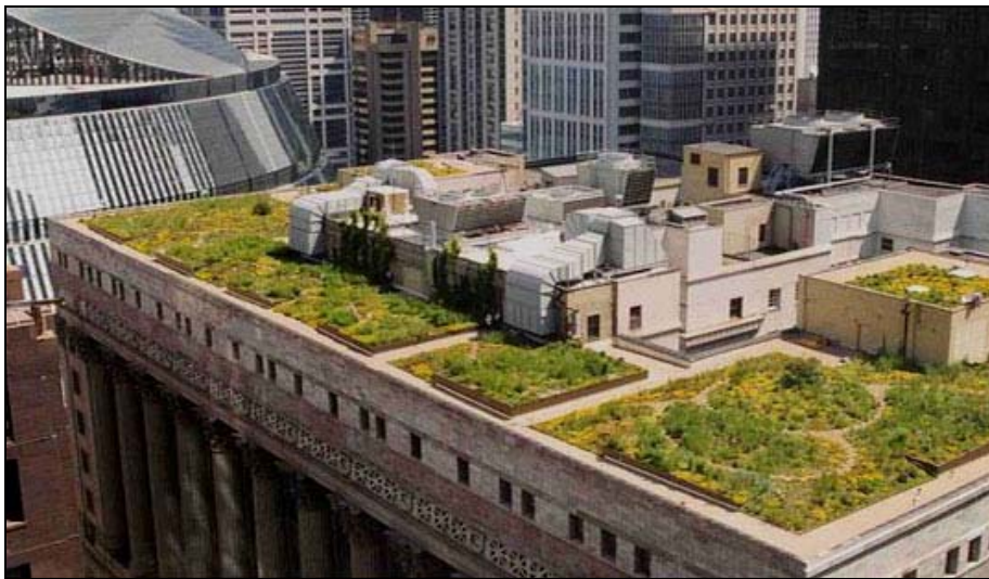
Figure 5.4: Green Roof on Chicago's City Hall
